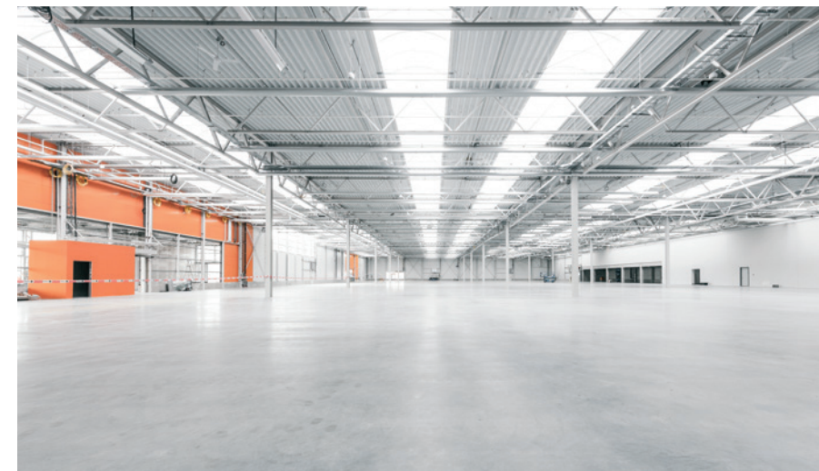
Top: Just an advert in February 2017, but by spring 2018 there will be a new HORNBAACH store here in Zwolle Middle: Colleagues discuss construction work in The Hague Bottom: Does it get any more beautiful than this? Top visibility thanks to light bands in the ceiling Left: The new store in Amsterdam shortly after its opening in February 2017
