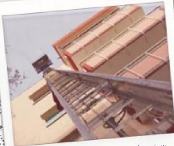
... and the goods hoist takes them up to the roof at maximum speed.
