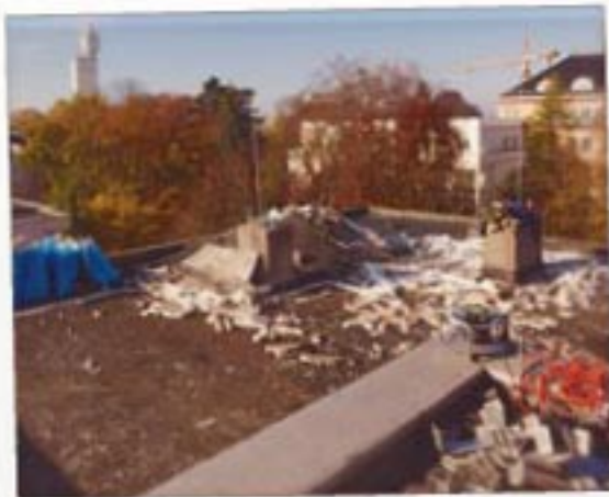
... but just a few hours later the roof is topless.
